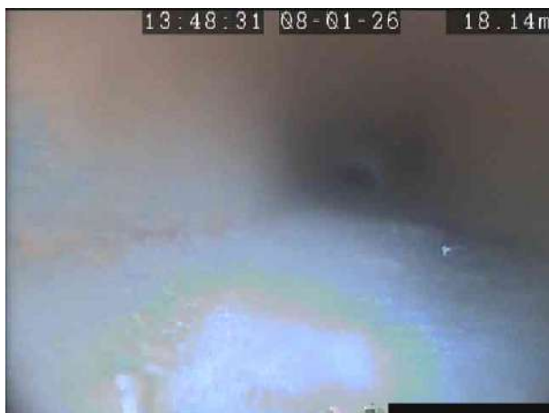
MH DX_899ca930-8445-46e7-aef0-201e26bab15e_20260113_16 2305_554.jpg, 00:01:06, 18.14 m Settled deposits, hard or compacted, 10% cross-sectional area loss
