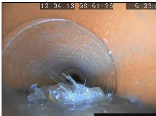
S5X_52bd08b9-b6b4-4cd2-ad4a-e77698905989_20260113_155342_968.jpg, 00:00:11, 0.47 m Settled deposits, coarse, 15% cross-sectional area loss, start
