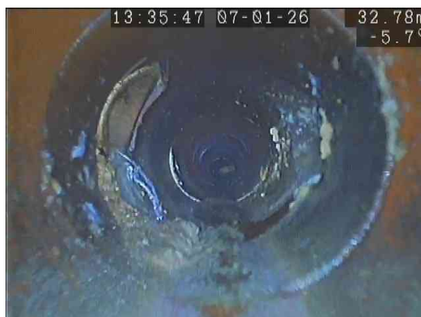
F9X_ca75f934-bbf3-4c72-8b8f-dea9d25fdc89_20260113_101937_686.jpg, 00:02:19, 32.86 m Connection other than junction at 10 o'clock, 150mm dia
