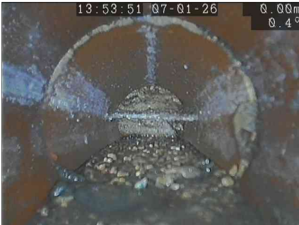
UTPX_c607b103-f1d8-406d-be87-3c6d7c140bbb_20260113_111002_082.jpg, 00:00:09, 0.01 m Settled deposits, coarse, 10% cross-sectional area loss
