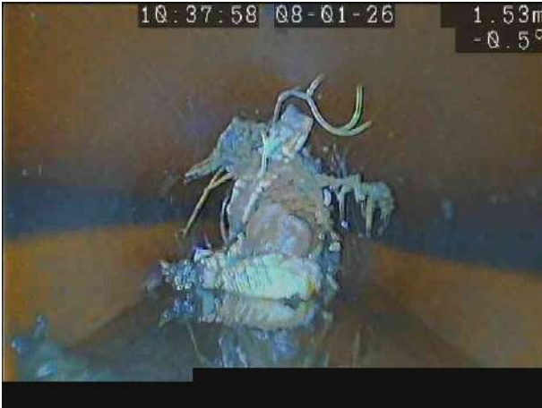
S10X_671d00d3-4286-4051-8b0f-f1f60877df32_20260113_13 2257_161.jpg, 00:00:25, 1.53 m Settled deposits, other, 70% cross-sectional area loss, Debris
