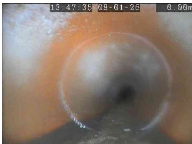
MH DX_e9422df4-dd7d-404b-b66d-610cfd9edc82_20260113_162 130_805.jpg, 00:00:10, 0.05 m Settled deposits, hard or compacted, 5% cross-sectional area loss, start
