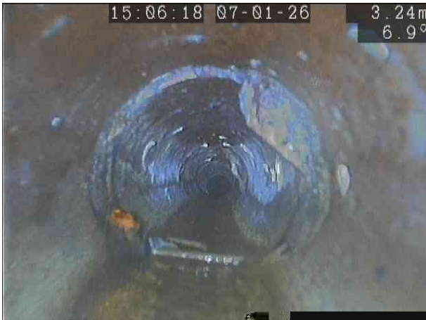
UTPX_6ca9bd6e-4dae-4868-8449-57a16b147dad_20260113_112935_007.jpg, 00:00:38, 3.31 m Settled deposits, hard or compacted at joint, 15% cross-sectional area loss
